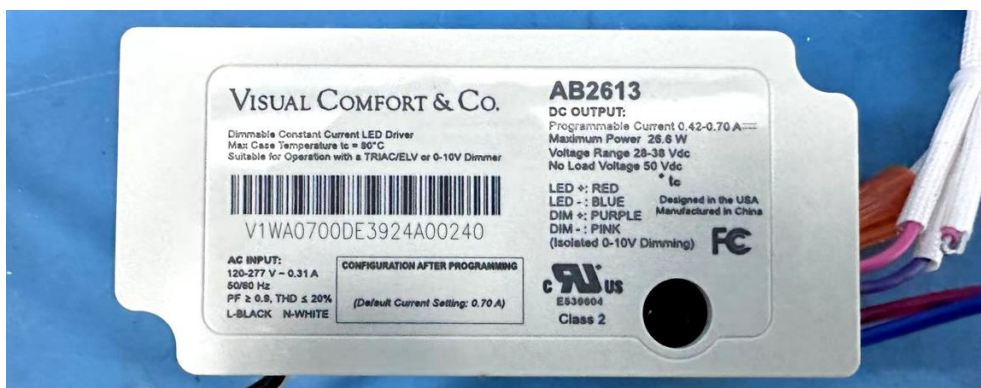
View of LED driver PSS30W-0700-38-VCC1 (AB2613)
